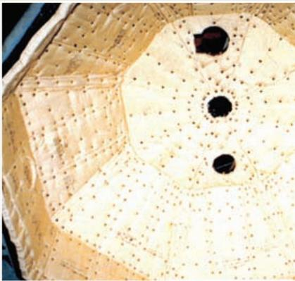
NUKON® blankets on the underside of a BWR RPV top bend "dog house."
