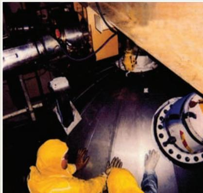
This shows the installation of NUKON® with MSG on a pressurized top head.
