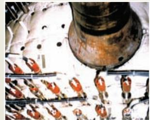
The NUKON® blankets on the bottom of head of this pressurizer can easily be removed for future inspection and reinstalled quickly without tools.
