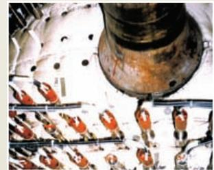
The NUKON® blankets on the bottom of head of this pressurizer can easily be removed for future inspection and reinstalled quickly without tools.
