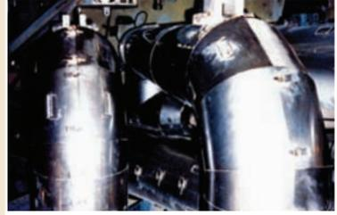
NUKON® pipe insulation installed inside the drywall of a BWR
