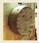
Semi-rigid RE/WRAP insulation cover,installed over man way on heated storage tank, guards against inadvertent worker contact with elevated temperatures
