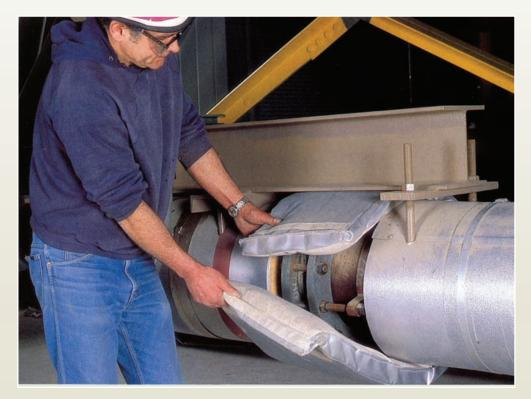
RE/WRAP Insulation blanket is applied over flanges in power plant ash-handling system where frequent service is required. Blankets are quickly removed when flanges require periodic maintenance, and can just as quickly be replaced. Adjacent piping, not requiring periodic maintenance, is covered with conventional insulation and aluminum jacketing. The system normally operates at 250°F but may experience temperature excursions above 600°F.
