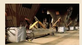
RE/WRAP insulation covers enclose ash-handling equipment arid controls beneath 144 precipitator hoppers at this coal-fired power plant. guarding operating personnel against contact with elevated temperatures. Insulation covers are of siliconeimpregnated fibrous glass fabric for wear resistance
