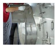
INSTALLATION/SUPERVISION OF REFLECTIVE METAL INSULATION (RMI)
