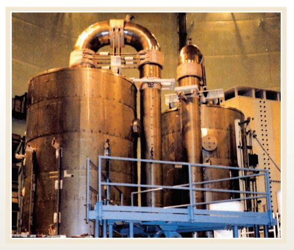
The NUKON® system is a nuclear containment thermal blanket insulation system.
