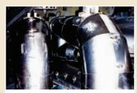
NUKON<sup>®</sup> pipe insulation installed inside the drywall of a BWR
