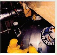
This shows the installation of NUKON<sup>®</sup> with MSG on a pressurized top bead.
