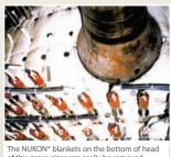
The NUKON® blankets on the bottom of head of this pressurizer can easily be removed for future inspection and reinstalled quickly without tools.
